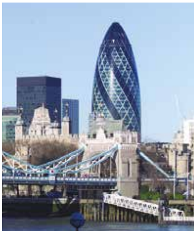
London's iconic "Gherkin" has 67 Aqua-Rex units on the electric water heaters.
